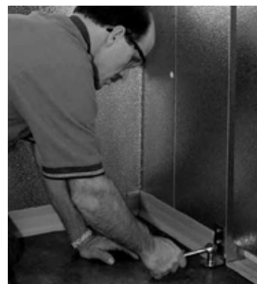
Attach slam brace with fastener provided
