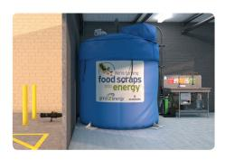
All Grind2Energy storage tanks include two tank vacuum breakers to allow air admittance during pump-outs, as well as a vent stack filter. For tanks housed indoors, powered ventilation (sold separately) is recommended to help mitigate/dissipate odor build-up in the tank.
